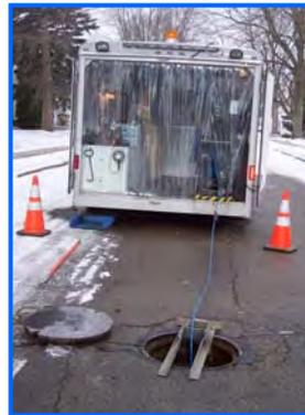
Televising sanitary lines identifies pipe in poor condition.
